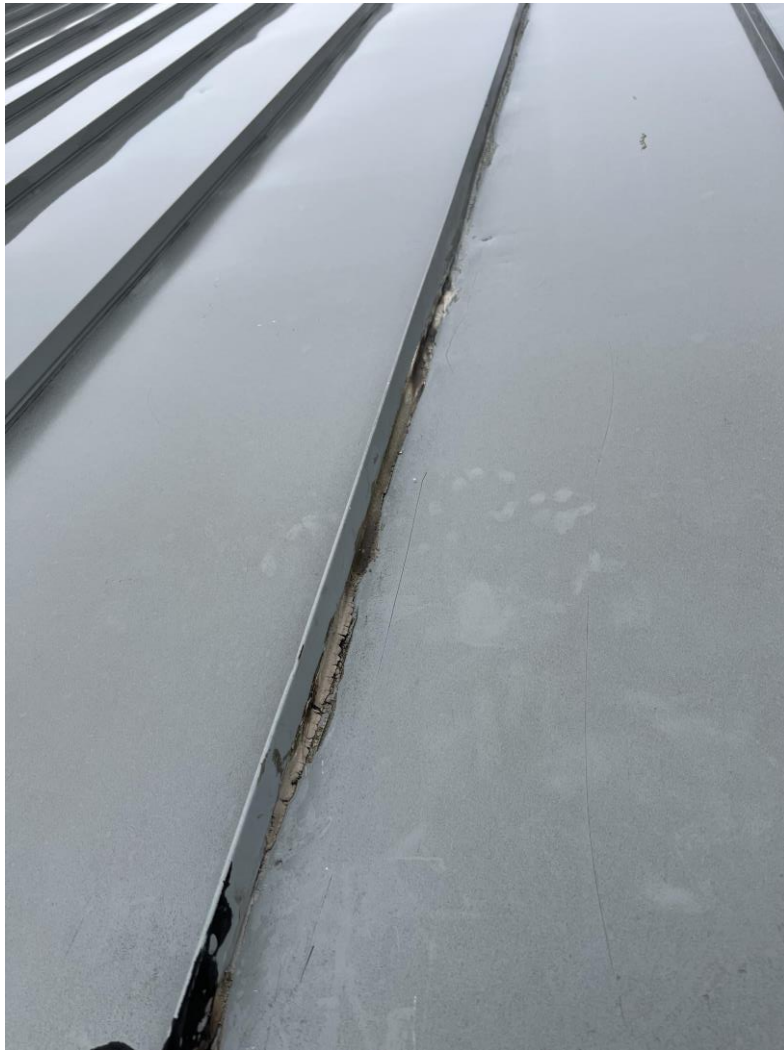
Panel is unstable; evidence of previous repairs made to stop leaks on the rib/seams
