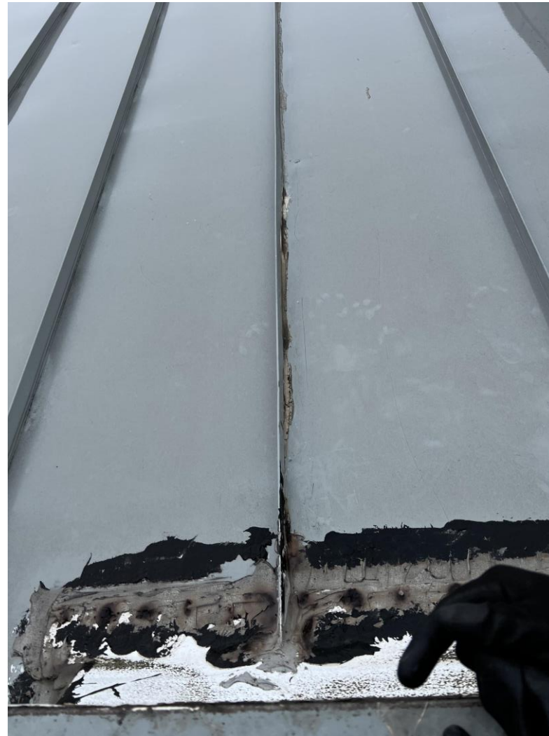
Roof hatch detail improperly flashed; previous repairs were made; as they leaked asphalt was used
