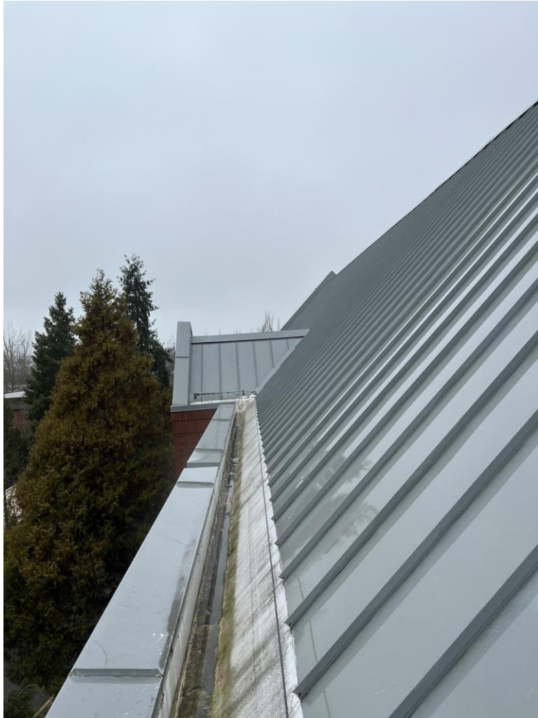
Eave detail; previous repairs were made on the EPDM (pictured on the right)
